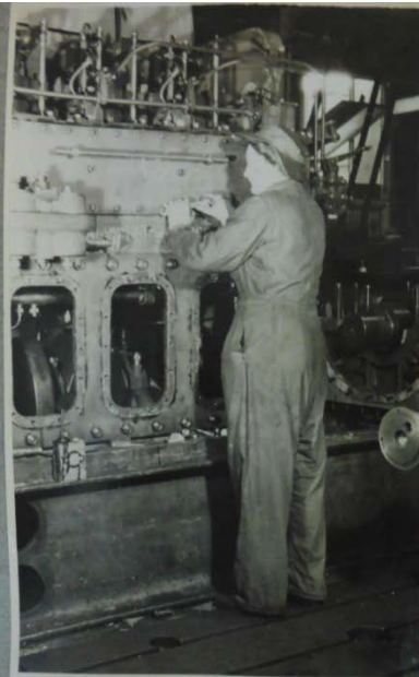
In the Main Erecting Shop, females are ass- isting skilled men on the fitting and erection of important Naval mach- inery. This worker is fitting the crankshaft door of a Diesel Engine
