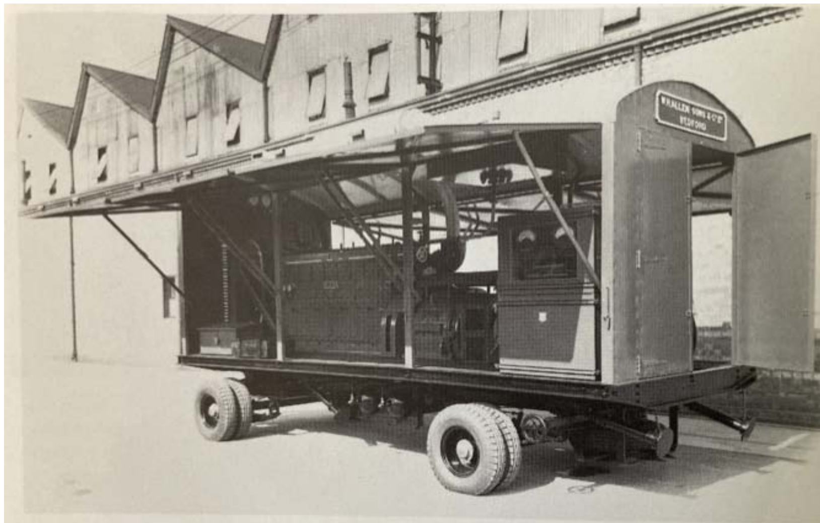
A portable emergency diesel generating set supplied to the Metropolitan Water Board during World War II.
