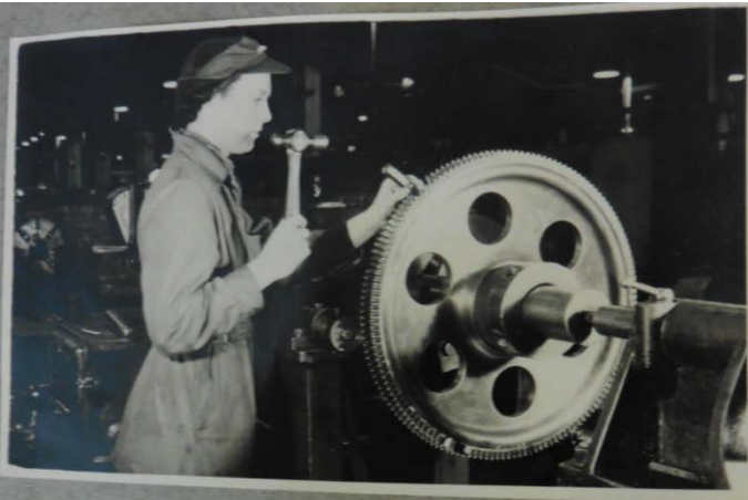
Blading the Rotor wheel of a Steam Turbine.
