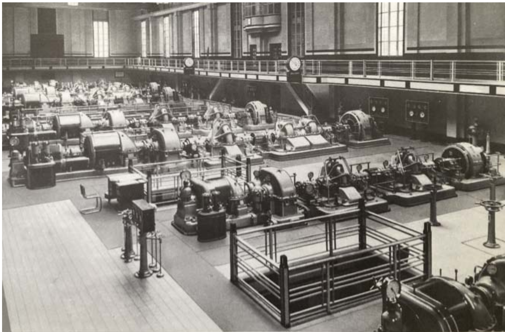
The machinery hall at the Metropolitan Water Board's Hampton Station showing the Allen turbine-driven pumping and generating units.
